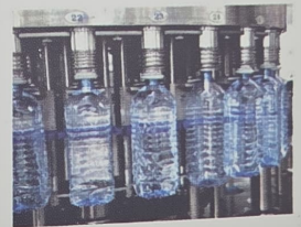
R O Water Plant
